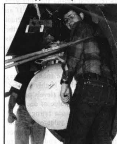
HANDS ON —TI's Mike Hill checks the antenna assembly inside the P-3 radome while working at San Clemente Island.
