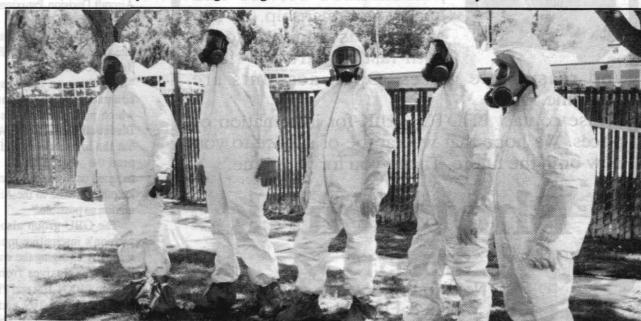
IT'S AN INVASION of the asbestos abatement preparation people. The "plastic" type suit, gloves and air filters protect the crew in case they encounter an asbestos spill and against the dust and debris they have to work in.
