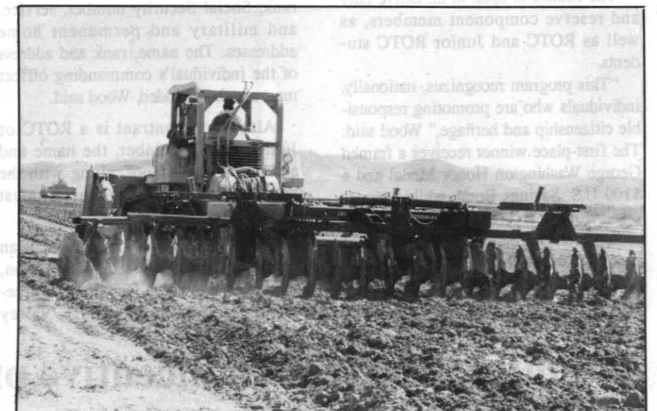
AIRCRAFT LANDING ZONE —Seabees use bull dozers and sheepfoot roller to compact the loose desert soil after a good old fashioned farm disk is used to mix soil and water for deeper compaction at Echo Range LZ.
