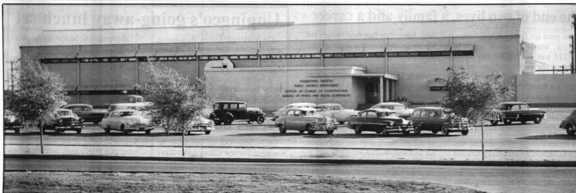
CIRCA 1953—Building 37 housed the OICC of the Bureau of Yards and Docks Contracts and the Engineering Division of the Public Works Department. TID file photo
