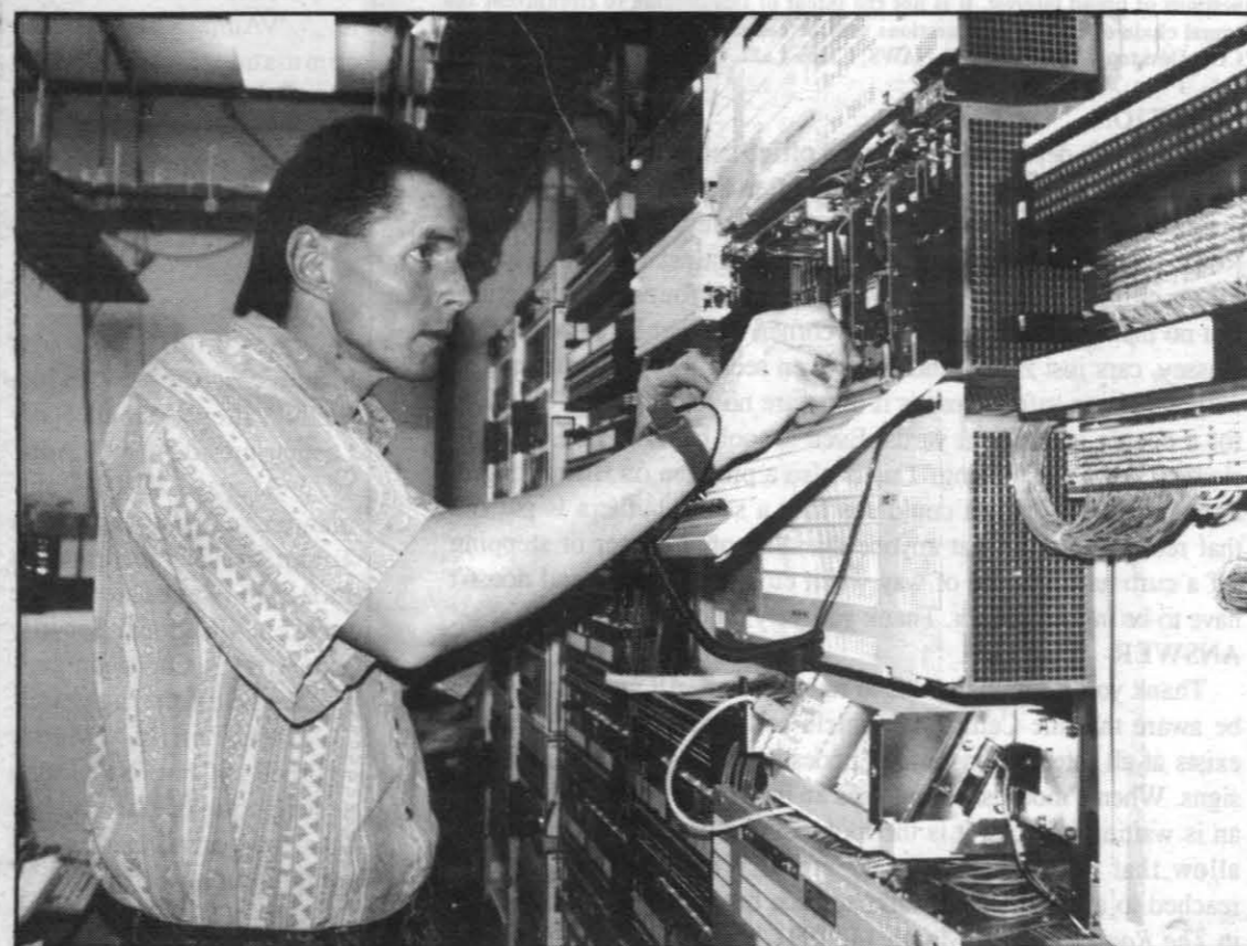
PREPARING for the cutover on Friday night, Brad Rollness, CASI switch engineer, adjusts the FMT150, which is the fiber optic transmission system connecting all China Lake sites into one system.
