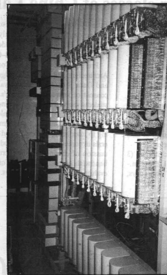
COMPARING THE NEW AGAINST THE OLD —Ruhl DeLaet, a CASI program engineer, looks at some of the new system's hardware, the Meridian SL-100 Switch. This switch replaces the outdated hardware such as the stepper switch, shown on the right. The new computerized system replaces technology that was developed more than 100 years ago.
