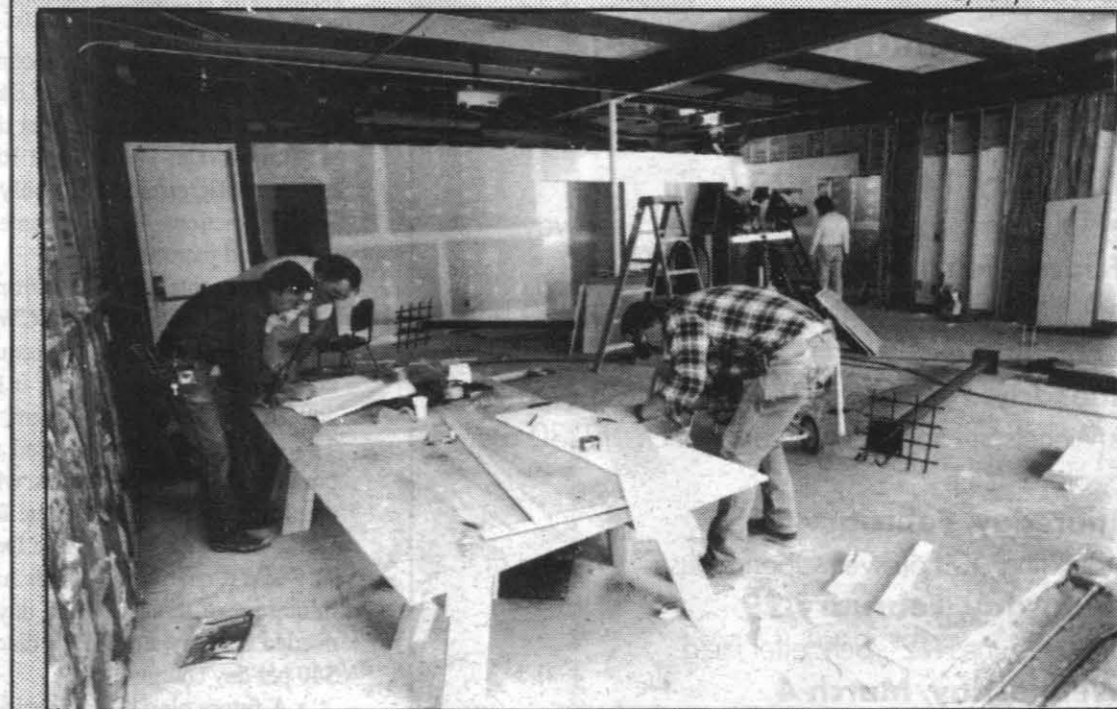
RENOVATION of the China Lake Conference Center (old Chief's Club) is on schedule and expected to be completed by the end of April. The effort will provide more efficient use of space and increase classified conference capabilities.
