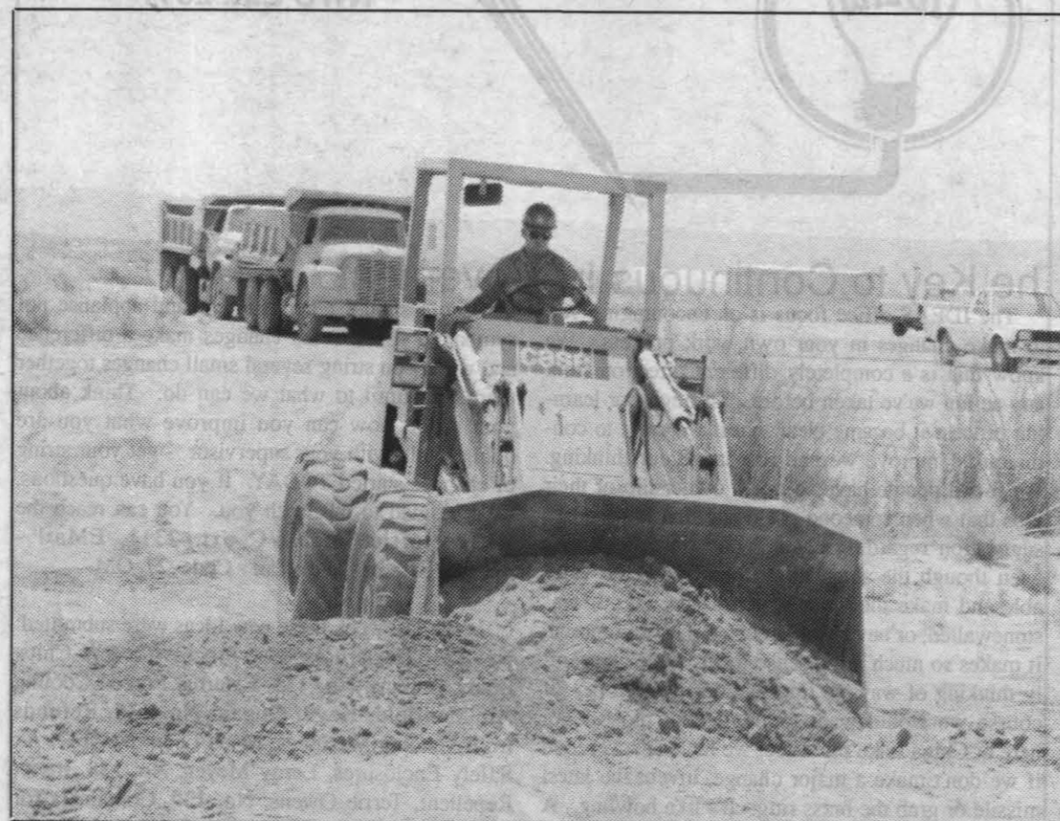
ROAD WORK--Reserve Seabees from RNMCB Detachment 0217 work near NWC's Thompson Lab.
