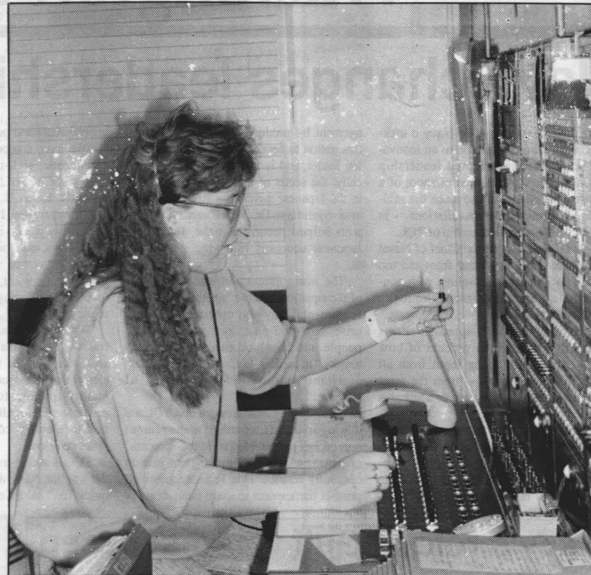
NUMBER PLEASE--Dina Durant, one of the few remaining telephone operators at the Naval Weapons Center, is ready to make a connection for a caller on the last known "cord board" switchboard known to be serving a community in California. Photo by PH3 Cary Brady
