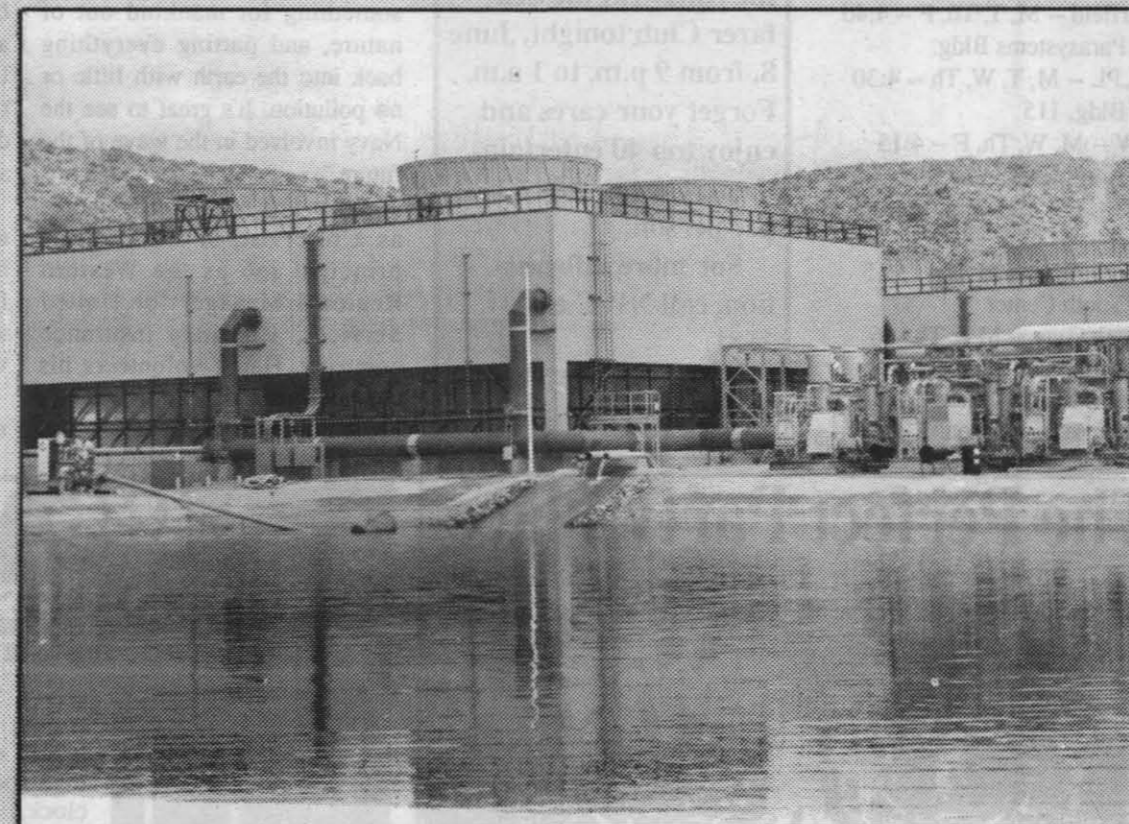
COOLING TOWERS-- When petroleum geologists visited the Coso Geothermal Plant, they saw huge cooling tower at work. The towers are an important part of the environmentally sound development of the geothermal resources at NWC.
