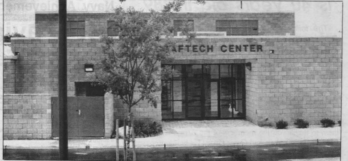
CRAFTECH FACILITY —This new building houses the Morale, Welfare and Recreation Division's Craftech Center. Capt. John Burt, NWC Commander, will snip the ribbon for the official grand opening this morning (Friday) at 10:30 a.m.
