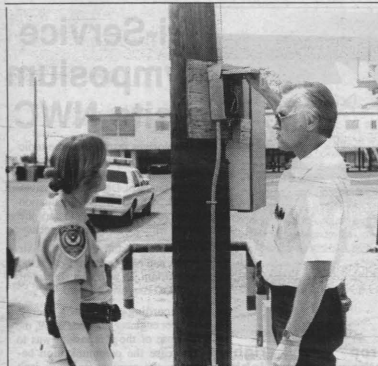
VANDALISM —Jim Bowen, head of Morale, Welfare & Recreation, inspects the damage done to an electrical box at Reardon Field with China Lake Police Officer Lisa Lyons. According to Bowen, someone apparently pried open the box and destroyed an electrical switch. "This kind of damage is costly," said Bowen, "resulting in higher prices for everyone. If you see or have seen anyone vandalizing NWC property, please report it immediately to the China Lake Police Division." Photo by PHAN Cary Brady
