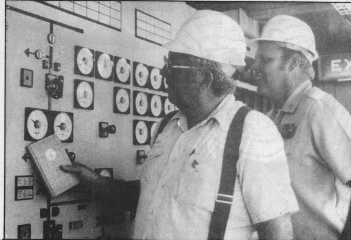
BIG MOMENT —Dr. Carl Austin and LCdr. Keith Haan of the Geothermal Program Office watch as the dials show that Power Plant One, Unit One is on-line and producing electricity
