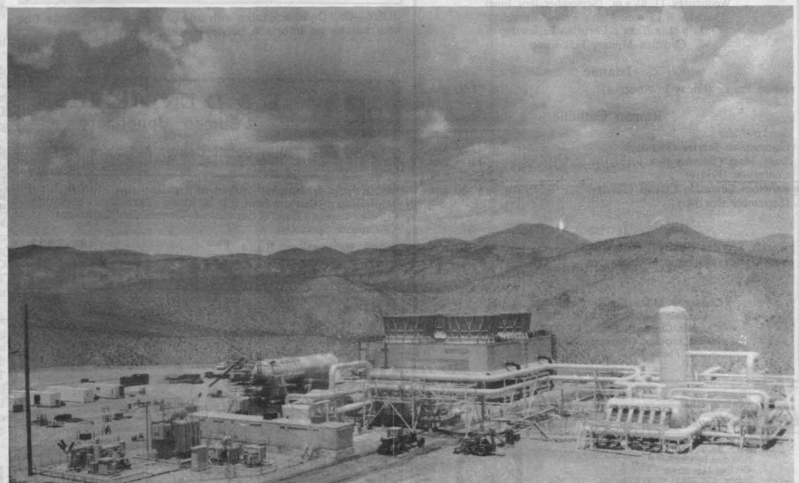
HUMMING ALONG — Power Plant One, Unit One of the Coso Geothermal Project went on-line last week, and now produces
