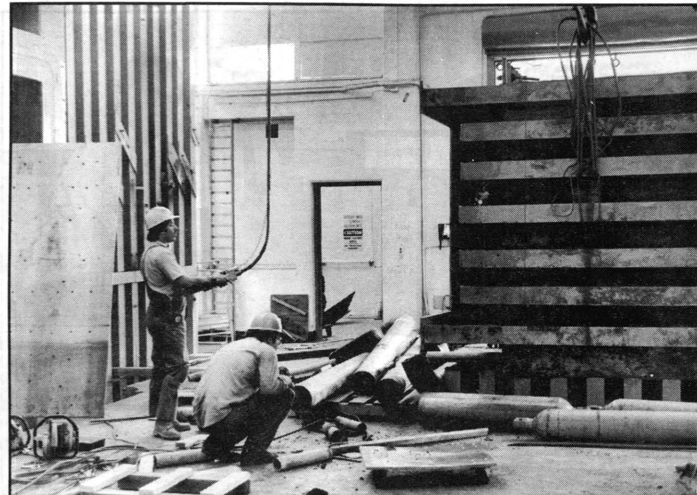
WILL IT FIT? — Workers check to see if they need to trim any more off a big section of the back of the environmental chamber so it can get through the door to Michelson Lab compound. (Yes, they had to trim another 14 inches — and clearance then was less than 2 inches a side.)
