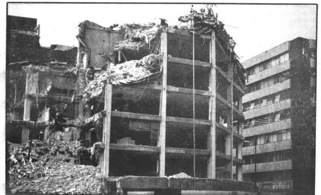
EARTHQUAKE DAMAGE — Mexico City is still recovering from the 1985 earthquake responsible for the damage in this photograph taken by Dr. Glenn Roquemore of NWC when he toured the city earlier this
