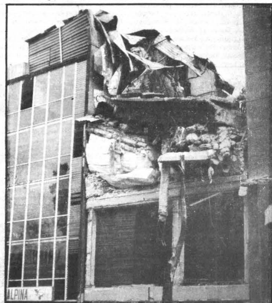
QUAKE DAMAGE — This is just one of many buildings damaged in Mexico City.
