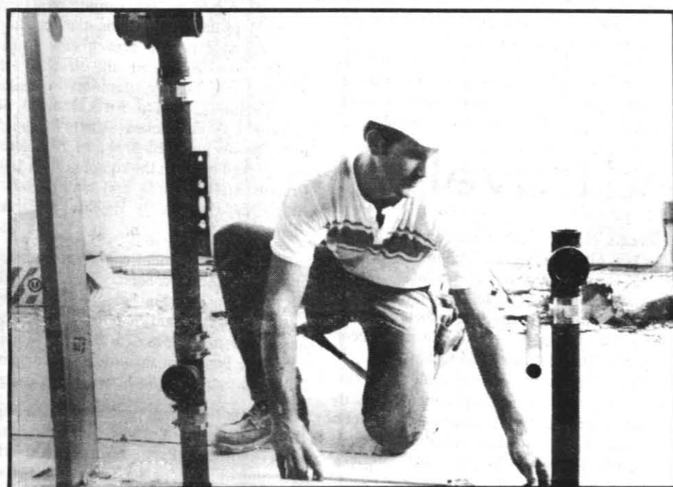
REHABILITATION WORK — Keith Cook, a plumber, is seen working on the NWC Training Center, now under going extension rehabilitation and remodeling. While the facility is under construction, for an estimated six months, Training Center personnel have been relocated to Building 02330, the white trailer behind the center and Chapel Annex 95, northwest of the white trailer. Phone numbers remain the same for training personnel. — Photo by PH2 Rick Moore
