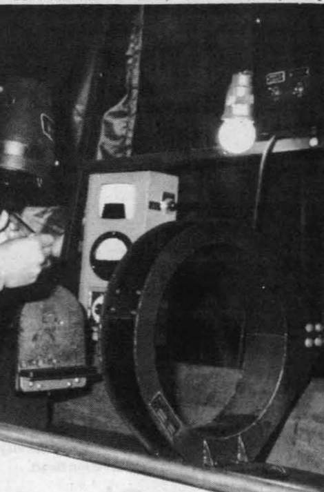
CAREFUL SCRUTINY — Performing one of the diversified procedures in the NDI shop, whose personnel look for damage in aircraft and ordnance, is Petty Officer Michael Judd. AD2 Judd is shown examining an F-4 speedbreak hydraulic piston during a magnetic particle inspection. — Photo by PHAN Greg Hogan
