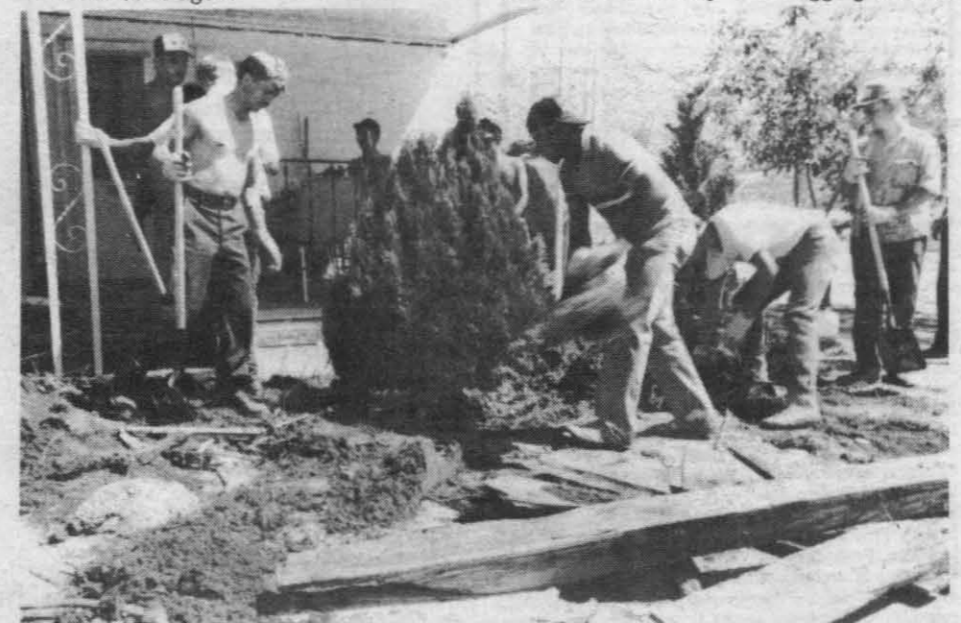
COOPERATIVE EFFORT — A group of volunteers from China Lake dig through the debris and dirt to determine whether the foundation on which this mobile home sits has been damaged by the sea of mud that engulfed it. — Photo by PHAN Greg Hogan
