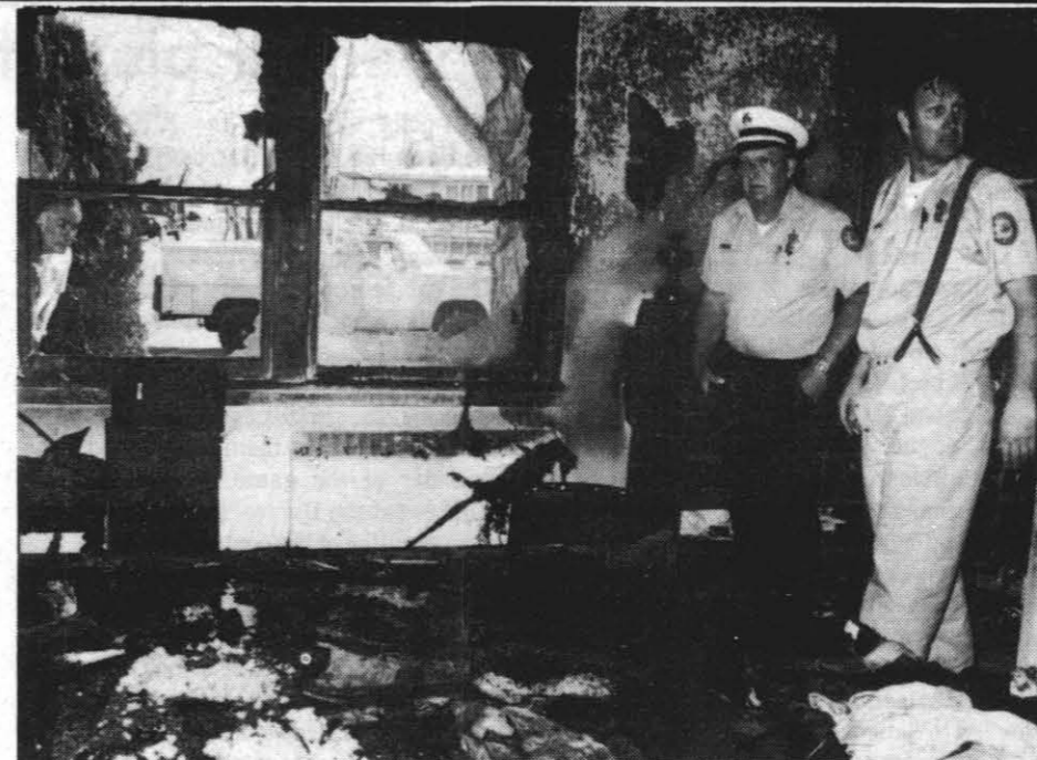
FIRE DAMAGE INSPECTED — Capt. Frank D. Holley (left), and Lt. Ray Ames of the China Lake Fire Division examine what's left of a bedroom after a fire in an old duplex located on Bard St. Thursday, Feb. 9. — Photo by PHAN Greg Hogan
