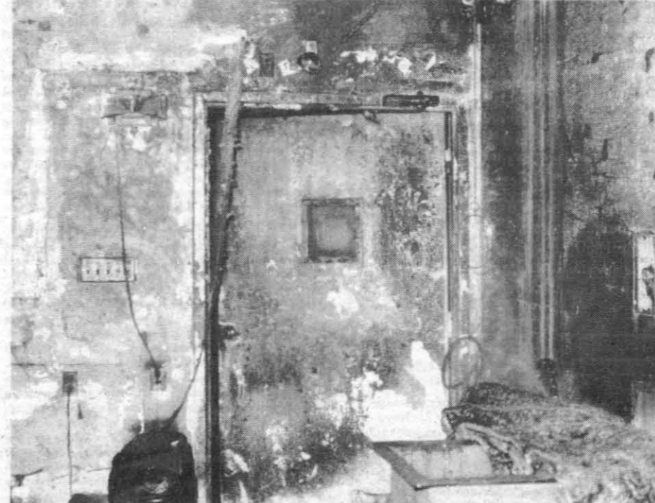
FOCUS OF ATTENTION — Efforts of those investigating the possible cause of the early Monday morning fire in the Michelson Laboratory Machine Shop complex is being concentrated on this room that housed equipment and chemicals used for tin/lead and copper plating of printed wiring boards. The fire door in center of photo served its function of keeping the blaze from spreading.
