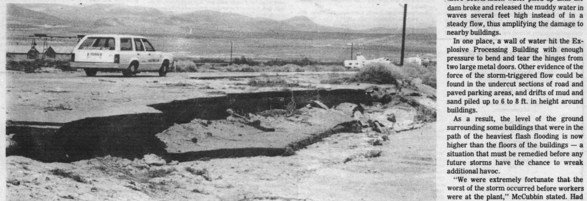
ROAD NETWORK DAMAGED — Roads leading to remote areas at Salt Wells, the northern ranges, and to Echo and Mojave B ranges on the south all show the effects of flash floods that covered an extensive area of the Indian Wells Valley.
