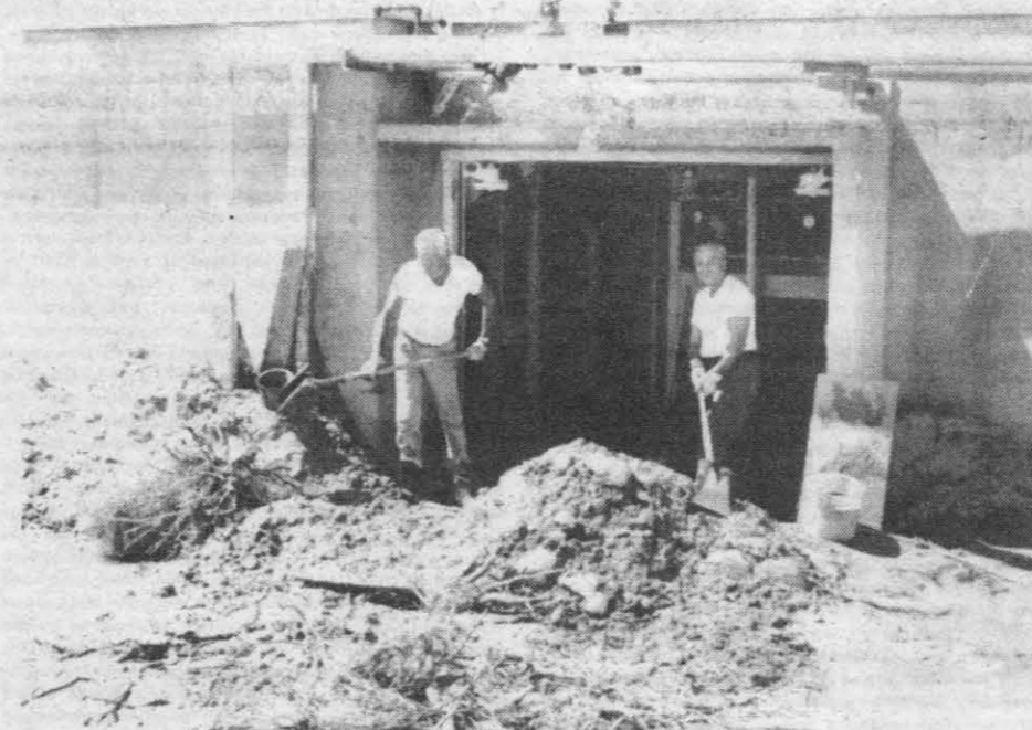
THE HARD WAY — If mechanized equipment suitable for ridding the interior of buildings of sand and mud is manufactured, it isn't available here. This leaves the task to workmen manning shovels. This building (No. 559) was one of those hardest hit in the Salt Wells area. When in operation, it is a melt cast explosive loading facility.
