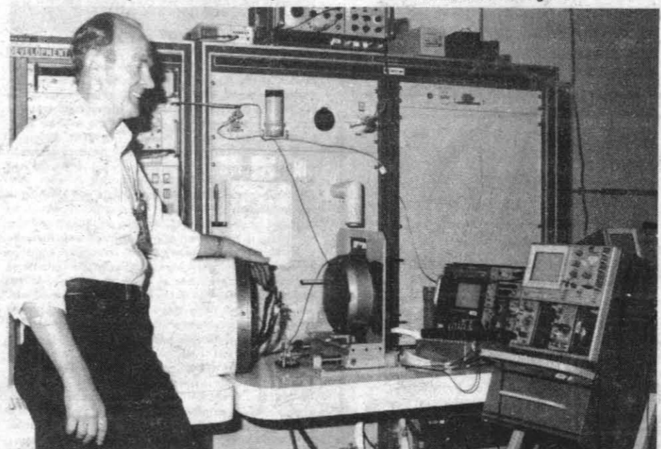
BIG HELP IN TEST WORK — H. J. Kirschsieper looks over the Mark 45 Engineering Development Test Set that is used for a laboratory check of modifications to the Mk 45 Mod 5 Target Detecting Device for the Standard Missile 2 weapon. Kirschsieper's outstanding efforts in the area of guided missile fuze system development earned him the NWC Technical Director's Award. — Photo by PH1 Benita Tetreault
