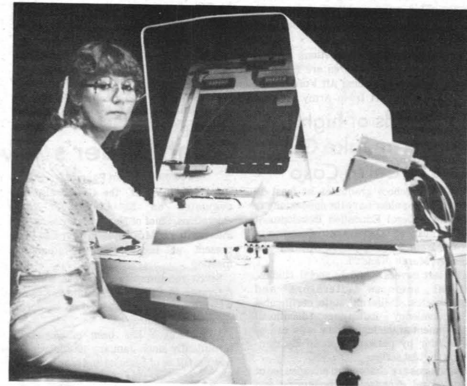
FILM READER — Kim Sturgeon is one of the employees for Computer Sciences Corp. in Ridgecrest who reads the film taken by cinetheodolite cameras during tests on the NWC ranges. The film reader is tied directly to a computer that is capable of advising the operator of errors in the film reading process, and also stores the data for later use for a multitude of purposes. — Photo by PH1 Benita Tretreault
