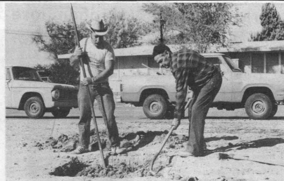
HARD AT WORK — Chuck Foster (l.) and Frank Brewer discover that caliche is as hard as cement as they dig a hole for the base of a merry-go-round that they then installed in a minipark and playground at Lauritsen Road and McIntire Street in the northern old duplex area. This is the third minipark and playground built under the self-help program by volunteer labor on weekends with materials furnished by the Housing Division.
