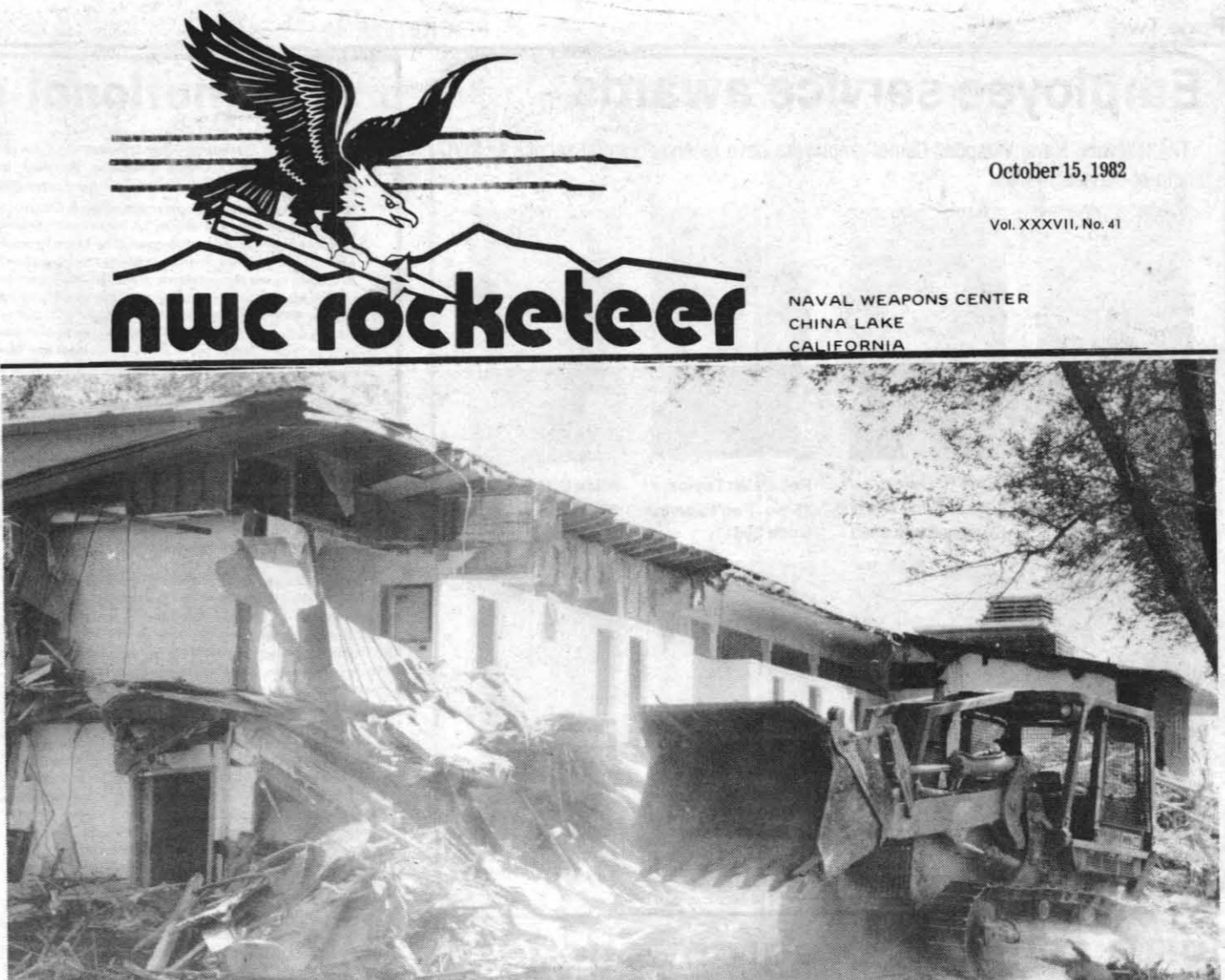
LANDMARK DISAPPEARS — Heavy equipment operated by workmen of the BEMAC Co. of North Hollywood ripped into and demolished the Housing Building — a structure that some old timers at China Lake may remember as their first quarters when it was used to house single men (barrack style). The wood-frame structure was "here today — gone tomorrow" as a powerful bulldozer ripped it apart, and then loaded the debris onto a truck so that it could be hauled away.
