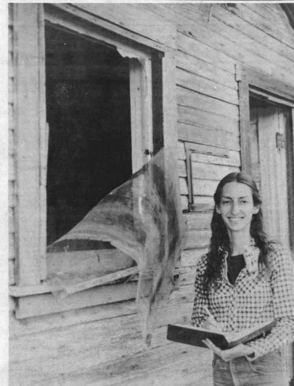
HOUSING INSPECTION — Wind, weather, and old age have caused this miner's cabin on the Center's north range area to deteriorate. Theresa Whitely, an archaeologist in the Environmental Branch of the Public Works Department, records its condition.
