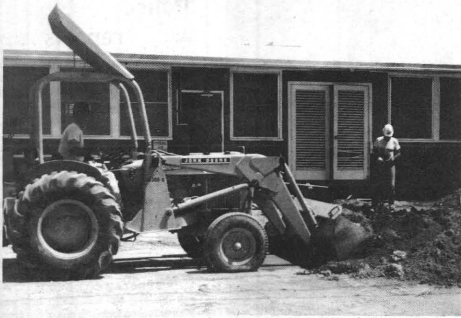
CHILDREN'S CENTER BUILDING RENOVATED — New steam vents have been installed in old Dormitory 6, which is now one of the buildings set aside for use by the Recreational Services Department's Children's Center. Sprinklers also are to be installed in compliance with fire safety regulations, and a playground area is to be added.
