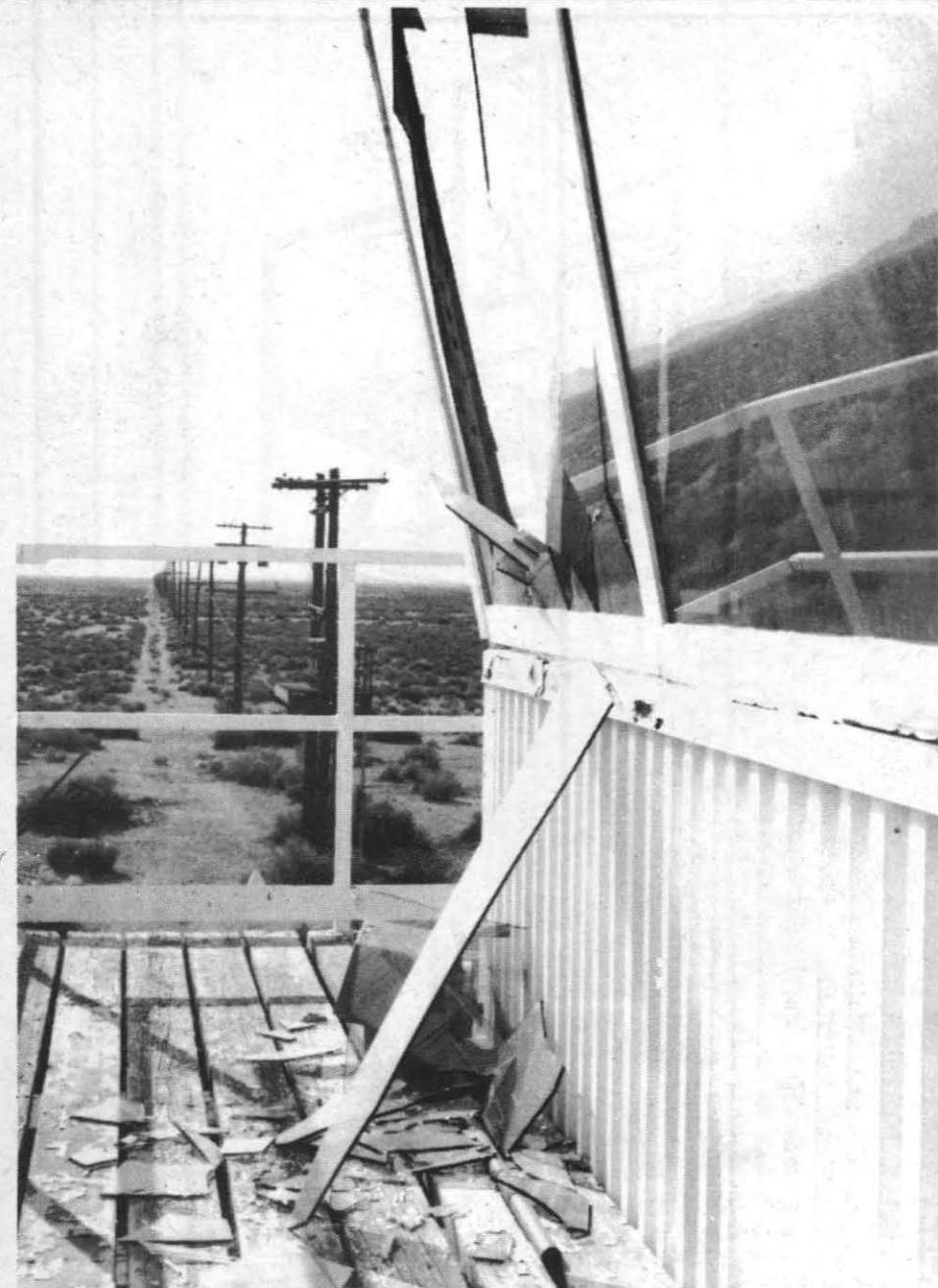
NATURE'S VANDALISM — East and west facing windows in Charlie Tower felt the full effect of last Sunday's earthquakes. Fortunately, no one was in the tower to be injured by the broken plate glass. Bookshelves in the tower spilled their contents, a fire extinguisher was knocked off the wall, and various free-standing items were knocked over by the force of the quakes. — Photo by Don Cornelius
