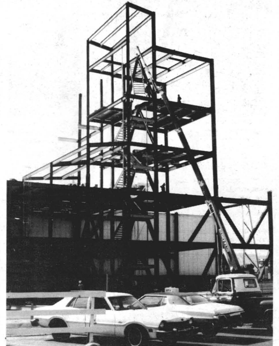
NEW BUILDING TAKES SHAPE — Steel girders, hoisted into place by a large crane, outline the shape of the Weapons System Support Facility that is being built at the east end of Hangar 3 at Armitage Airfield. Most of the underground utilities were installed before workmen began the steel work, which is now about 70 percent complete. Steel decking will follow, and then the lightweight concrete floors for the five-story structure will be poured. — Photo by Jon Partin
