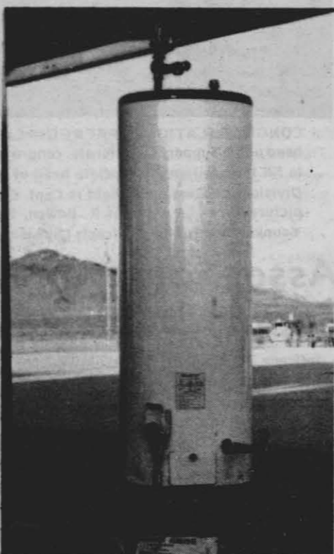
EFFICIENT OPERATION — Hot water heaters tend to be very wasteful of either natural gas or electricity, but this one, part of the Center's exhibit at the Energy Fair, uses the sun to bring 40 gallons of water up to the temperatures desired to handle a family's household needs.
