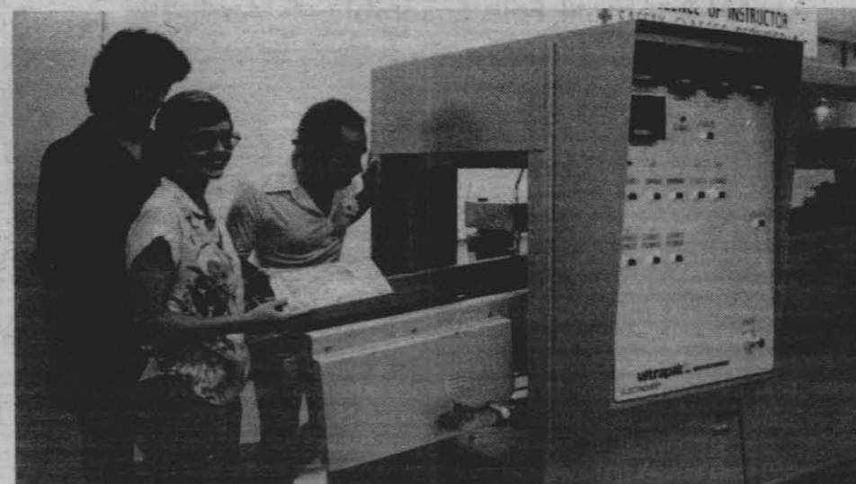
MOVE TOWARD AUTOMATION — Three employees of the Engineering Department's Soldering Technology Branch (1-r.) Kathi Johnson, Donna Sanger and Bill Vuono demonstrate how (if it was actually in use) a printed circuit board is fed into the wave soldering machine — one of the pieces of equipment that eventually will lend itself to totally automated production of printed circuit assemblies. When it is in operation, a conveyor system on the wave solder machine moves the printed circuit board across a wave of molten solder that solders all of the components on the board at one time. — Photo by PH2 Benita Tetreault
