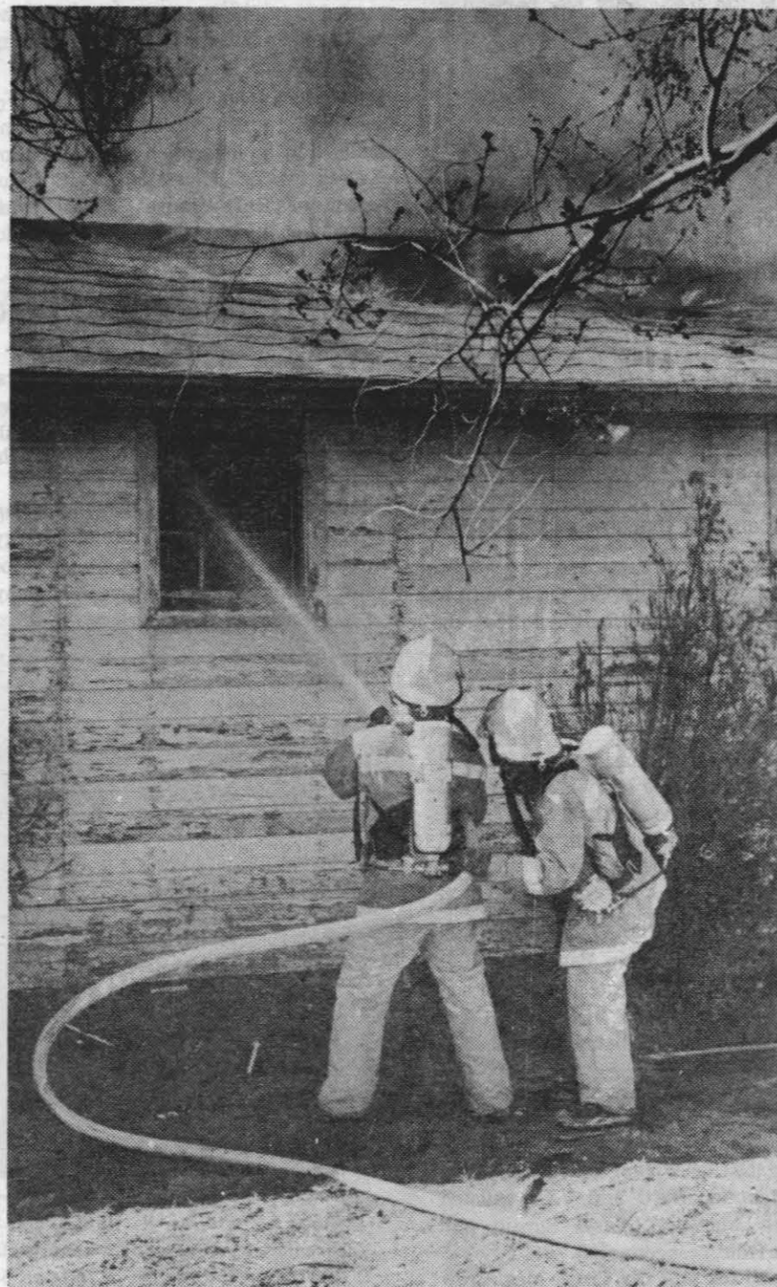
EXTERIOR ATTACK ON FIRE — The smoldering roof signals the likelihood that it could burst into flames at any time. For this reason, fire suppression efforts are carried on from outside by directing a stream of water through a window.
