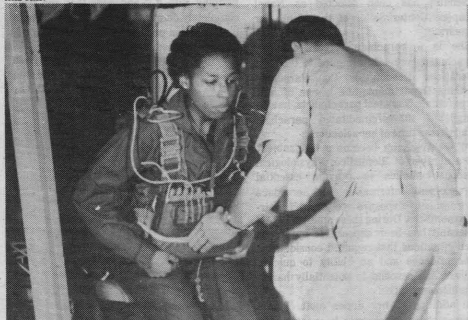
PRE-TEST CHECKUP — HM3 Constance Terrell is carefully fitted with test equipment by Lt. John Gilbert of the Biomedical Branch in the Parachute Systems Department before she begins ripcord tests.
