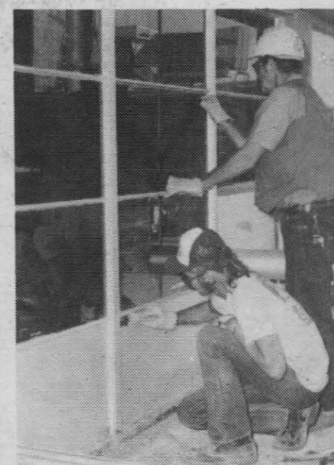
LETTING LIGHT IN — During the recent Energy Awareness walk-through, Richard Smith, a visual information specialist in Code 388, called attention to windows in one room of Michelson Laboratory that had been covered with opaque paint for an optical experiment years ago. By scraping the paint from these windows, the amount of electric light needed in the room could be markedly reduced. Natural light now shines in that room.
