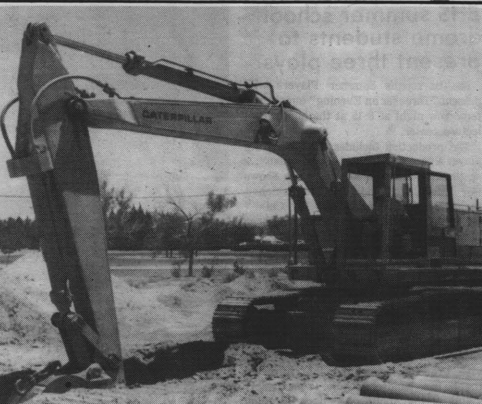
SEWER LINE DUG - Heavy equipment in operation last Friday not far from the traffic circle gives indication of the progress that has been made on work that is underway to improve the Naval Weapons Center's industrial-domestic sewer system. As this photo was shot, a trench was being dug for an 8-in. sewer main that will run from the Public Works compound to Michelson Laboratory. Another sewer line will be extended from the laboratory to industrial waste ponds located at the intersection of Lauritsen and Pole Line Rd.
