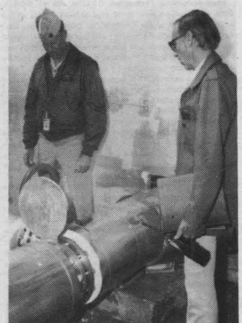
SHUTOFFS — Capt. Haff and Dr. Lind examine valves in the 10-in. pipe through which LNG is spilled for tests. The new LNG Spill facility has been constructed with all feasible safety factors because of the extremely hazardous materials being tested.
