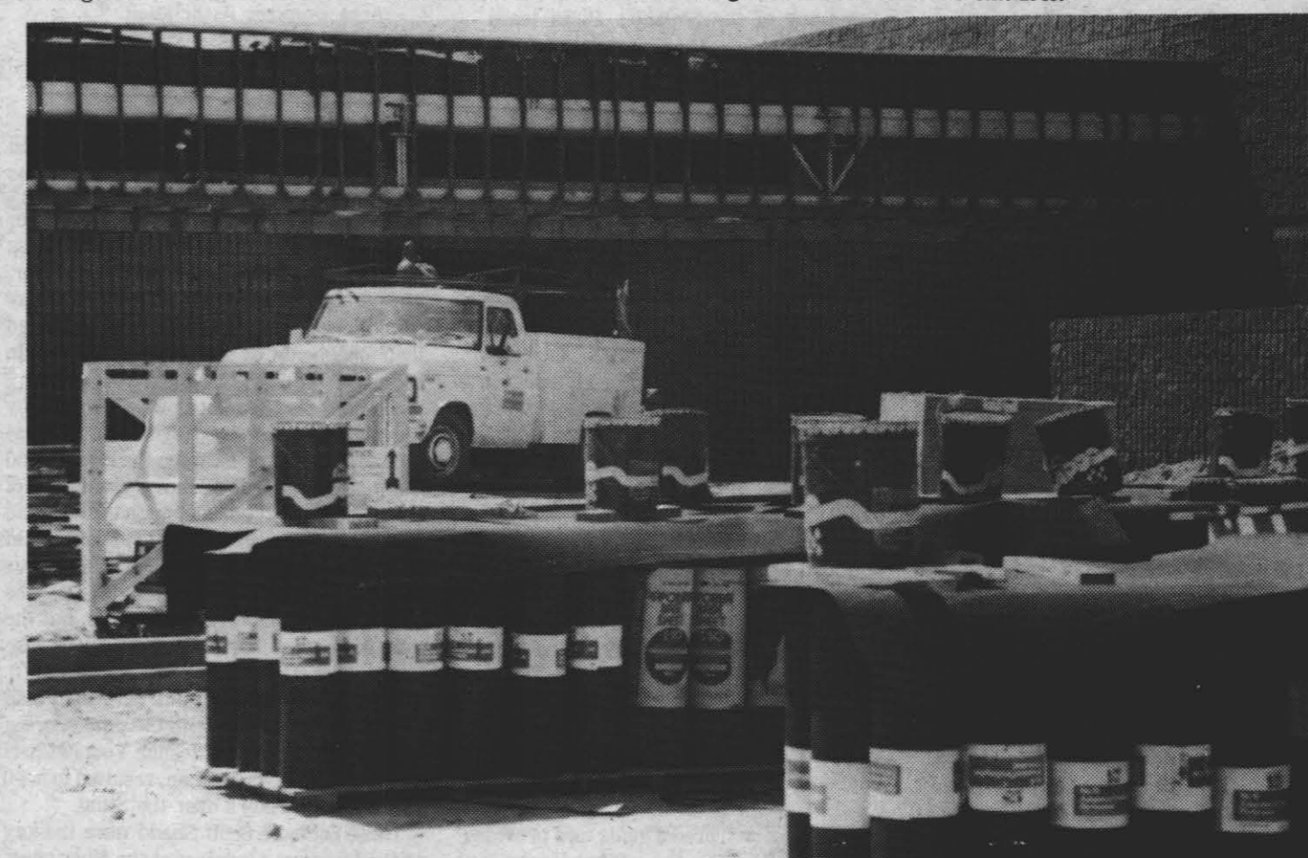
BUILDING WORK PROGRESSES — From the outside, the Range Control Center building now looks very much like it will when it is completed in early November, but a considerable amount of work still remains to be done inside. Rolls of roofing
