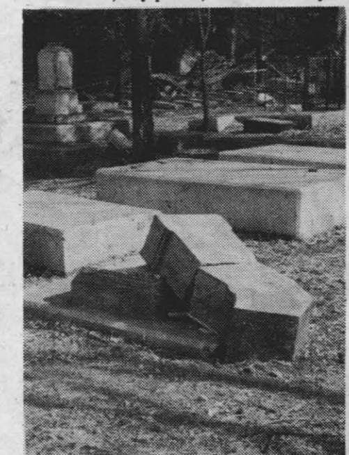
SHAKEN LOOSE — The toppled tombstone following the Nicaraguan quake of 1972 shows dramatically what happens with any structure that is not firmly bolted to a foundation. Mobile homes are especially susceptible to slippage from their concrete pier foundations.
