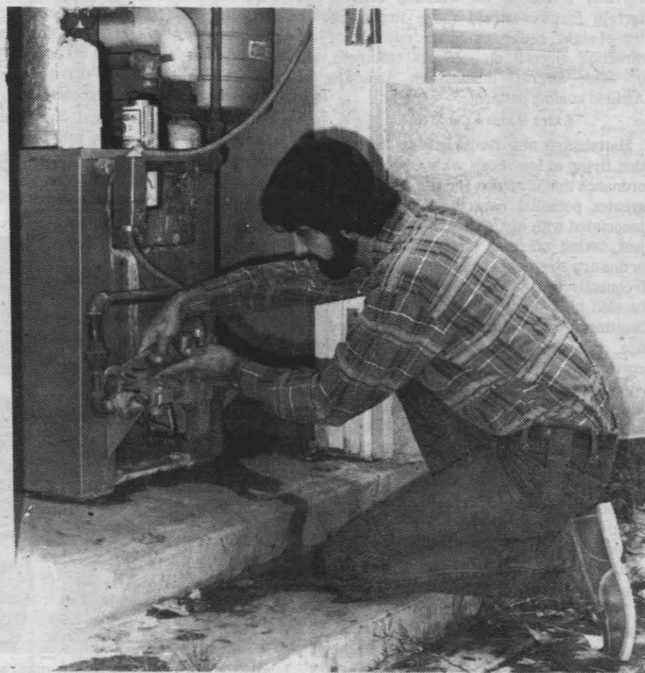
DRIP, DRIP, DRIP — Richard Brown, a plumber from the pipe shop, works with a residential heating system that is sputtering and leaking. Plumbers are among the Public Works Department personnel who are on duty 24 hours a day to meet industrial and residential emergencies.
