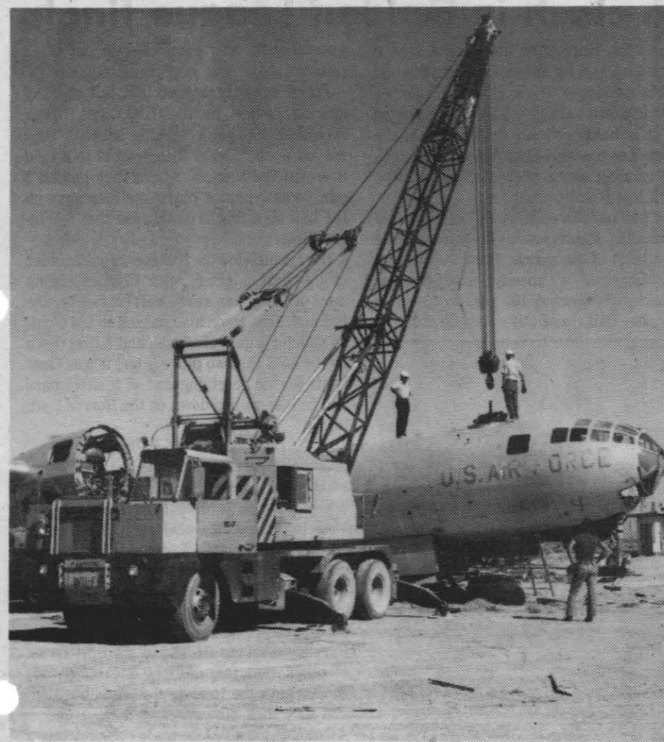
A LARGE CRANE is used to extract a turret from another aircraft in the scrapyard for eventual installation in the restored B-29 destined for England.
