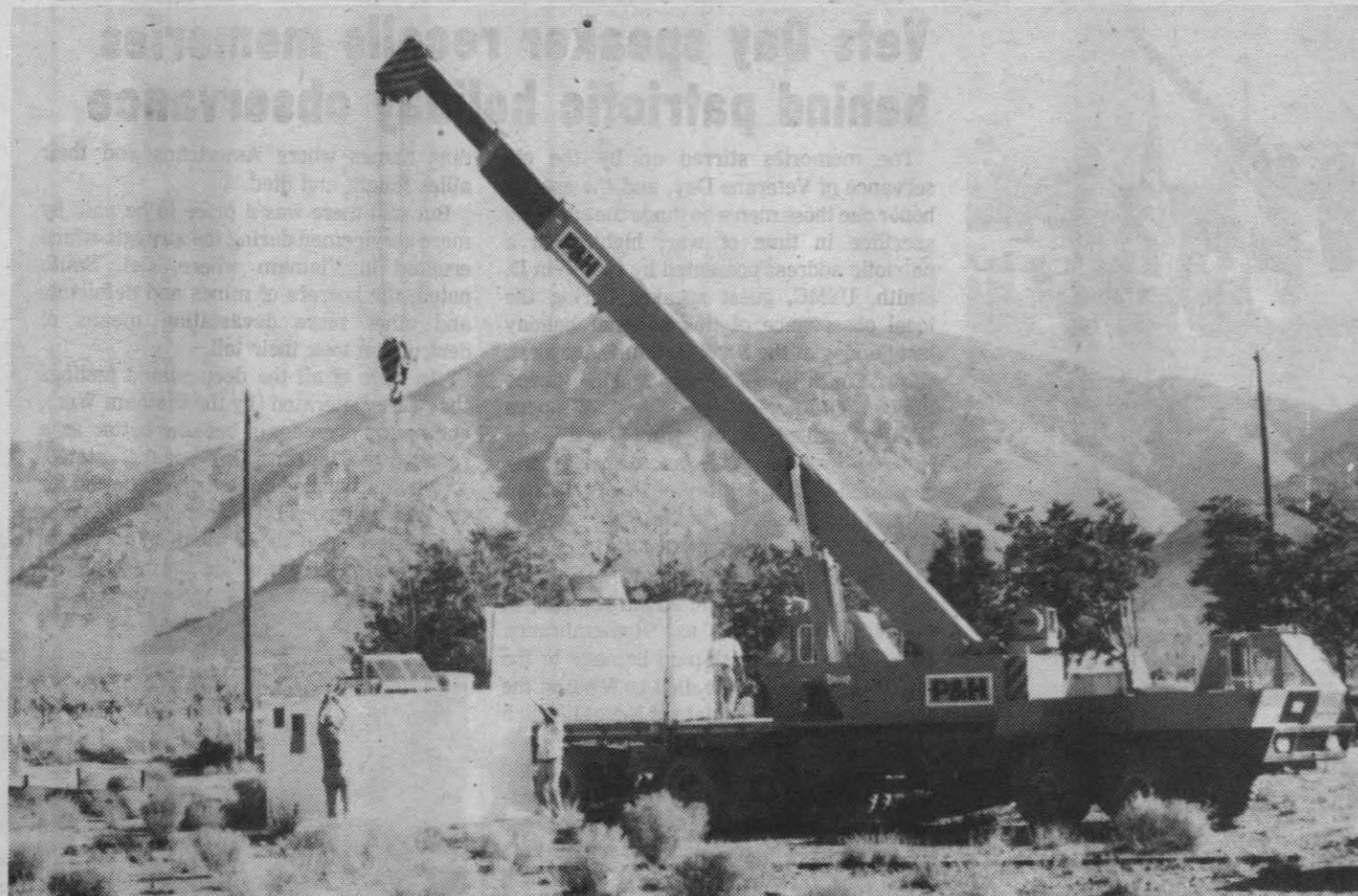
GENTLY NOW! — A giant crane gently lowers a shelter unit containing an emergency radio at the site of Junction Ranch in NWC's northern range area. Three of these radios are now operational at remote sites. The photovoltaic panels visible on top
