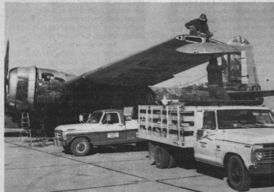
THE LAST STRUCTURAL problem to be remedied was replacement of the outer wing on the port side—a precaution deemed necessary when corrosion was found. As this photo was being taken, the outer tip of the wing was being fastened in place.
