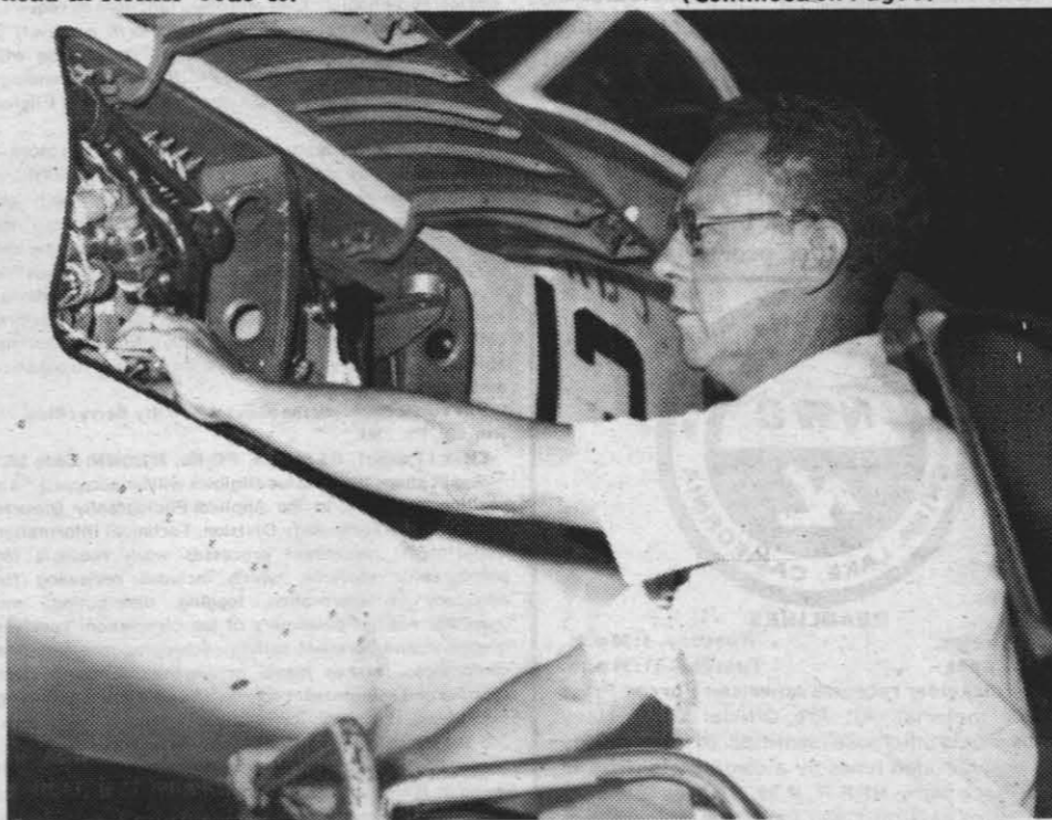
EQUIPMENT CHECKED PRIOR TO TEST — Carl Burkey inspects Angle Rate Bombing System (ARBS) equipment in the nose section of an A-4M Skyhawk aircraft prior to a test. Burkey, who is a system design engineer in the Systems Development Department's A-4M/AV-8 Project Office, this week received the Technical Director's Award in recognition of his key role in the development of ARBS. — Photo by Ron Allen
