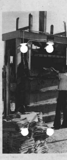
BALING - Newspapers collected are. sorted (to remove cardboard or magazines) and then baled for ease in handling. As they are baled, they are sprinkled with water to help cut down on dust (up to 5 percent of weight of newspapers collected for resale can be water). Jim Fath gets set to toss a load in the baler
