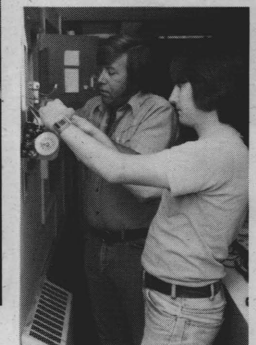
SETTING THE CLOCK — Bill Burum and Tom Lystrup install a time clock to control the evaporative coolers for one of the work areas in Building 981. The men have installed time clocks in three Public Works complex buildings and have also installed demand switches so that coolers can be turned off in areas in which no one is working.
