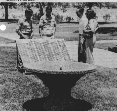
AN UNUSUAL ATTRACTION set up outside the Community Center was this solar energy powered water fountain. The sun's rays striking an array of silicon wafer cells that absorb energy produced the power needed to make the water flow.
