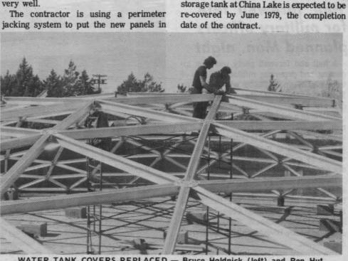
WATER TANK COVERS REPLACED - Bruce Holdnick (left) and Ron Hutchinson, ironworkers from the Temcor Corporation in Torrance, Calif., work on the dome of the underground water storage tank located near the traffic circle at the Naval Weapons Center. The wooden covers to four NWC reservoirs are being replaced with aluminum domes at a cost of \$685,000.
