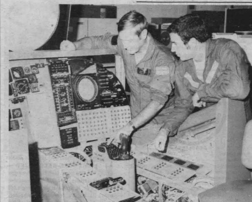
SIMULATED COCKPIT — Cdr. Andy Miller (left), deputy manager of the A-6 Software Support Activity, and Lcdr. Dabbieri demonstrate some of the features of the A-6 Simulation Facility which is used to duplicate actual flight and target conditions when validating A-6E (TRAM) Intruder computer program tapes.
