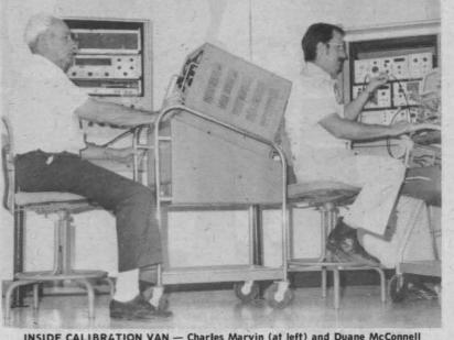
are the operators of the Engineering Department's new on-site calibration van. As this photo was taken, Marvin was operating an electronic counter to calibrate a singal generator. McConnell is using an oscilloscope calibration system.
