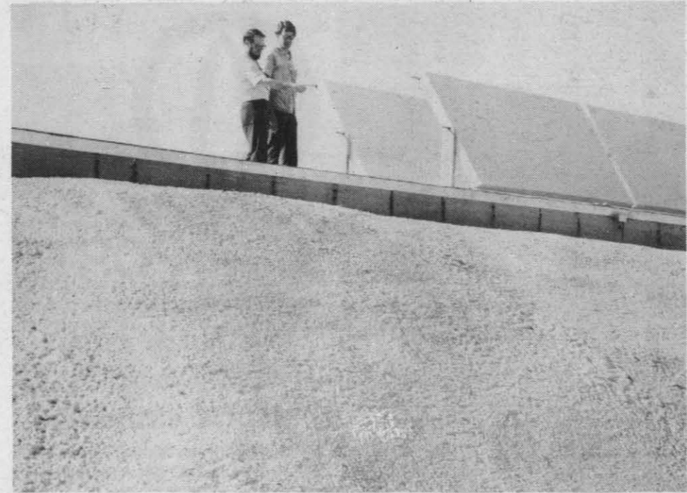
LOW ENERGY STRUCTURE TEST CELL —The mass of gunite-covered earth piled against the revetment in which the LES test cell is being built appears to dwarf the two men standing on its roof near the louvers, which open above a glass-covered, enclosed central area called "atrium." —Photo by Alan Fry
