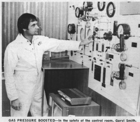
shown at the control panel of bench-scale pyrolysis gas purification and polymerization system, prepares to boost the pressure of purified gases before they go into the polymerizer.
