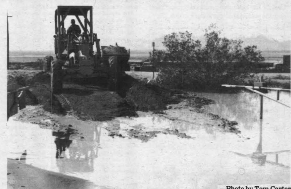
AFTERMATH OF STORM — A massive dose of work lies ahead for employees of the Public Works Department's Transportation Division as they carry out tasks necessary to repair NWC range area roads that were damaged by the recent rainstorms. This photo was taken near G range at the turnout to Burro Canyon. —Photo by Tom Carter
