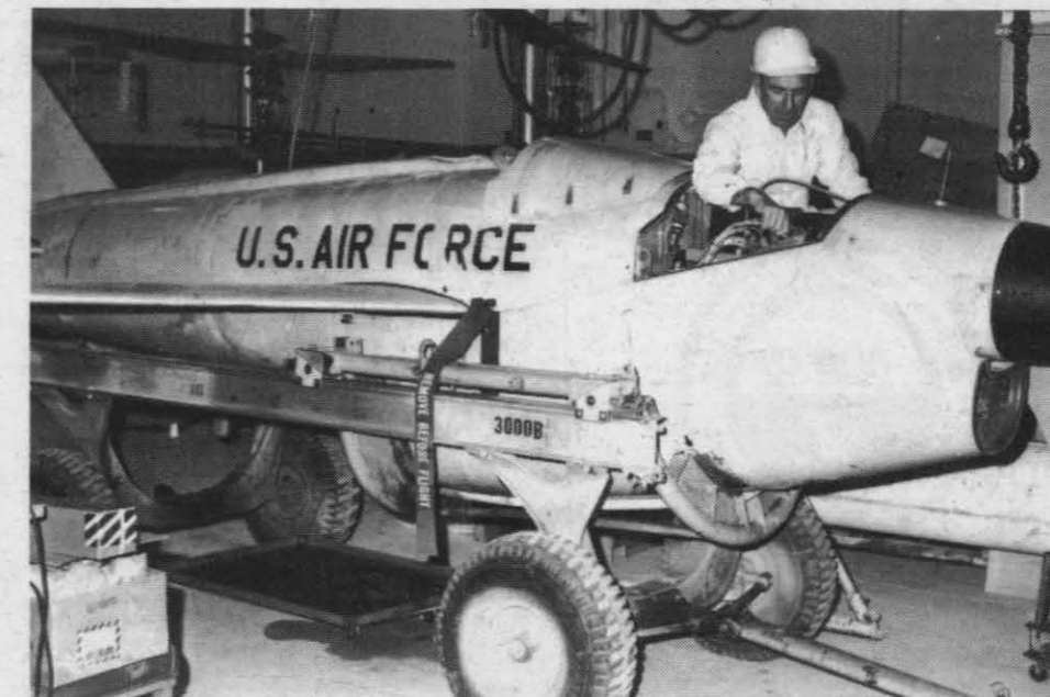
DRONE USED IN MISSILE TESTS — Charles Darrah, an engineering technician in the Targets Division of the Aircraft Department, checks the swivel release for the main parachute on a Firebee drone similar to those used here during the interface testing of the Sidewinder AIM-9L missile with the weapon system of the U.S. Air Force F-15 Eagle aircraft. The Firebee, which is 23 ft. long and has a wingspan of 13 ft., is capable of reaching a speed of 500 mph and can be operated at a maximum altitude of 60,000 ft. —Photo by Ron Allen
