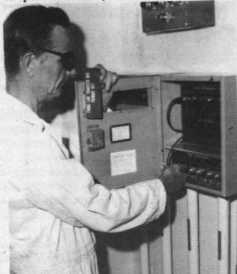
SAFETY FIRST — Charles Mitchell, an Explosive Technology Branch firing officer, checks firing line connections at a safety transfer panel.
