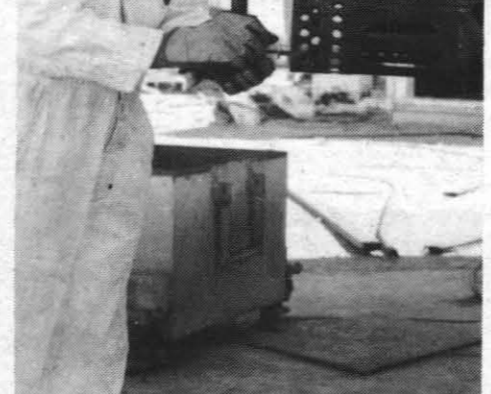
PREPARING TO FIRE — George Campbell, range engineer at K-2, prepares to boreight the business end of the Lightweight Gun Pod, which was mounted on a firing test stand.
