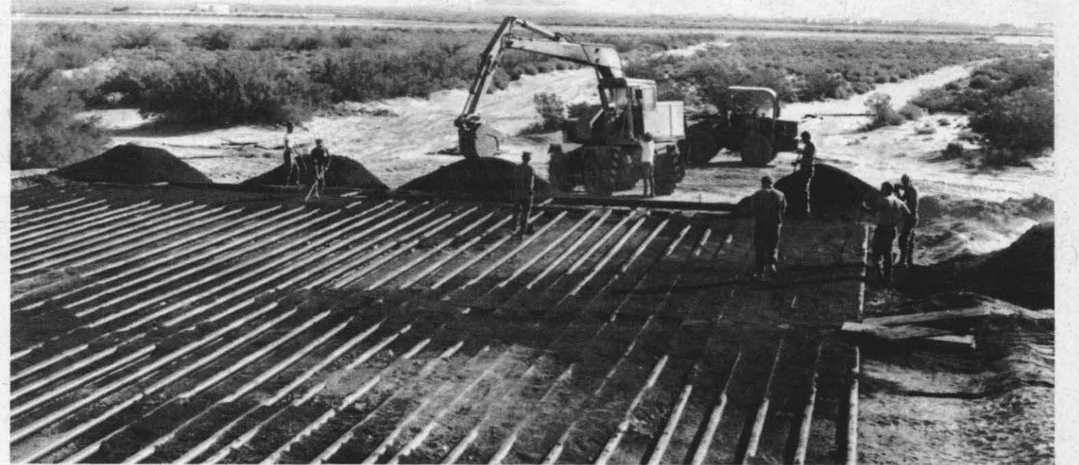
WORK AND MORE WORK — This bird's-eye-view of the solar heating project site at the NAF swimming pool gives some idea of the extent of work facing local and out-of-town Seabees as they tackled the job of laying down 150 tons of asphalt mix (or 8,000 sq. ft.) in just two days in order to provide insulation for the radiator-like grid of water lines in which well water is heated.
